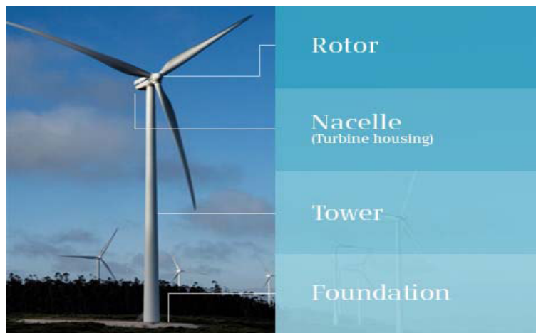
Figure 6: Anatomy of a Wind Turbine Generator
